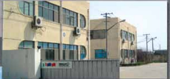
Shanghai Plant (PRC)
