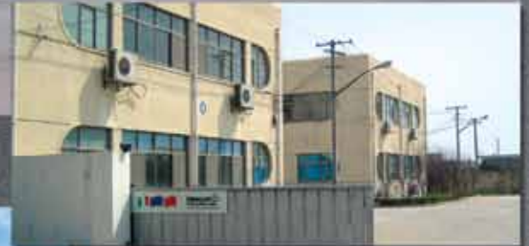
Shanghai Plant (PRC)
