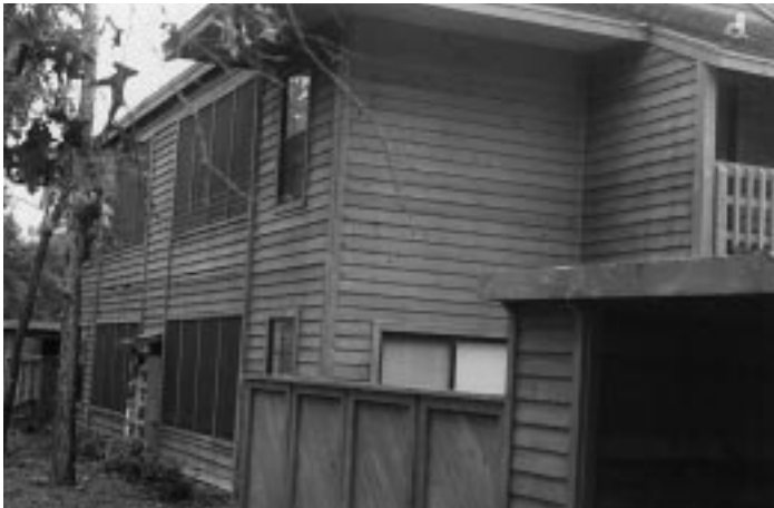
After Cedar siding restoration
