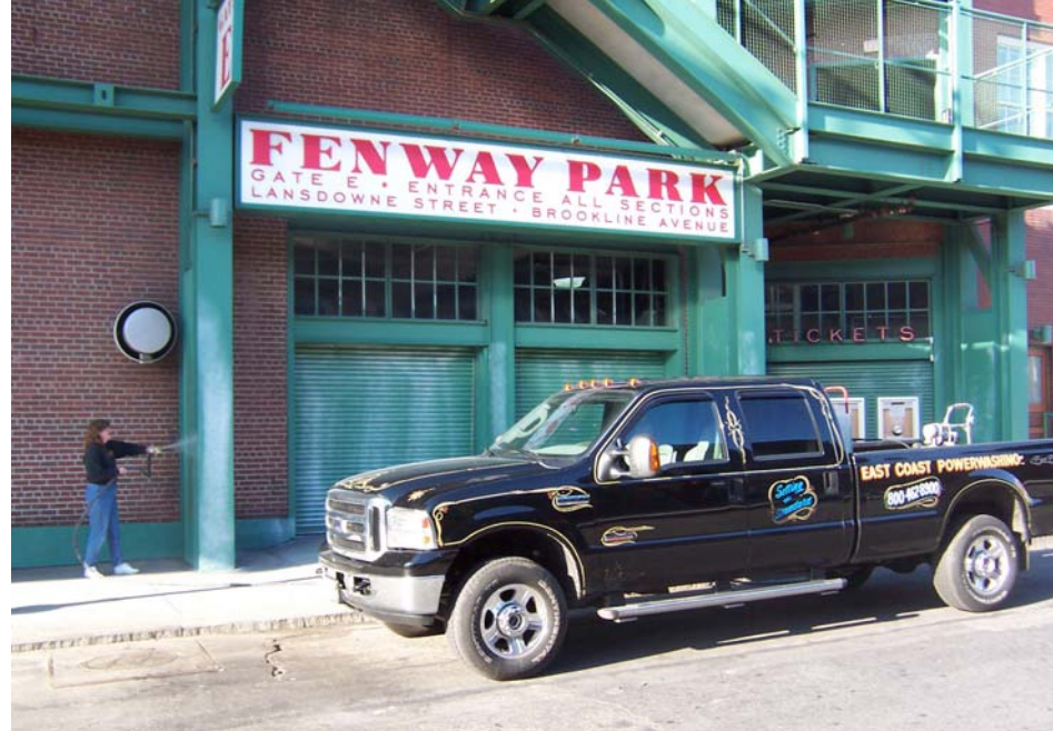
Spraying Fenway Park with a coating to protect it from graffiti
