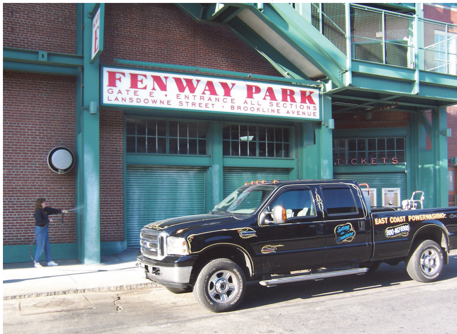
Spraying Fenway Park with a coating to protect it from graffiti
